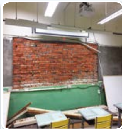
拆除黑板後露出紅磚牆
